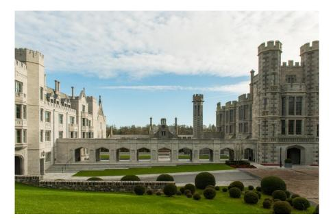
The locally sourced limestone used for the colonnade and West Wing is a near match to the original limestone while other new façade features and materials complement the existing, albeit with a character and finishes that are distinctly more modern and restrained. New window frames match the existing in
